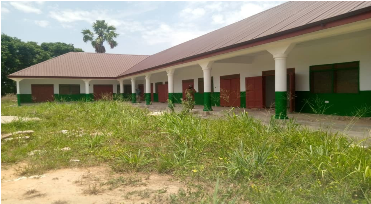
Current state of the project
