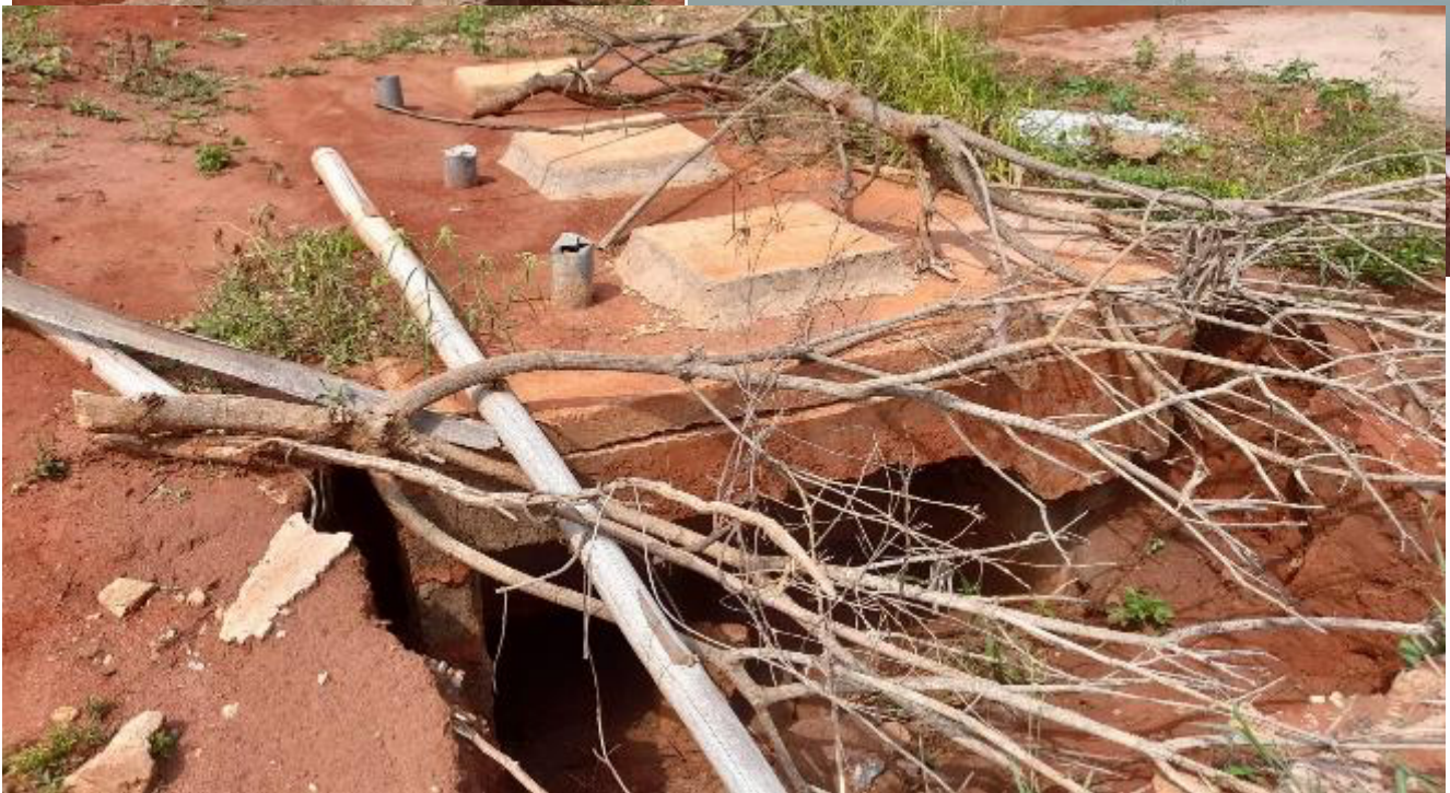
Uncompleted Tank stand
