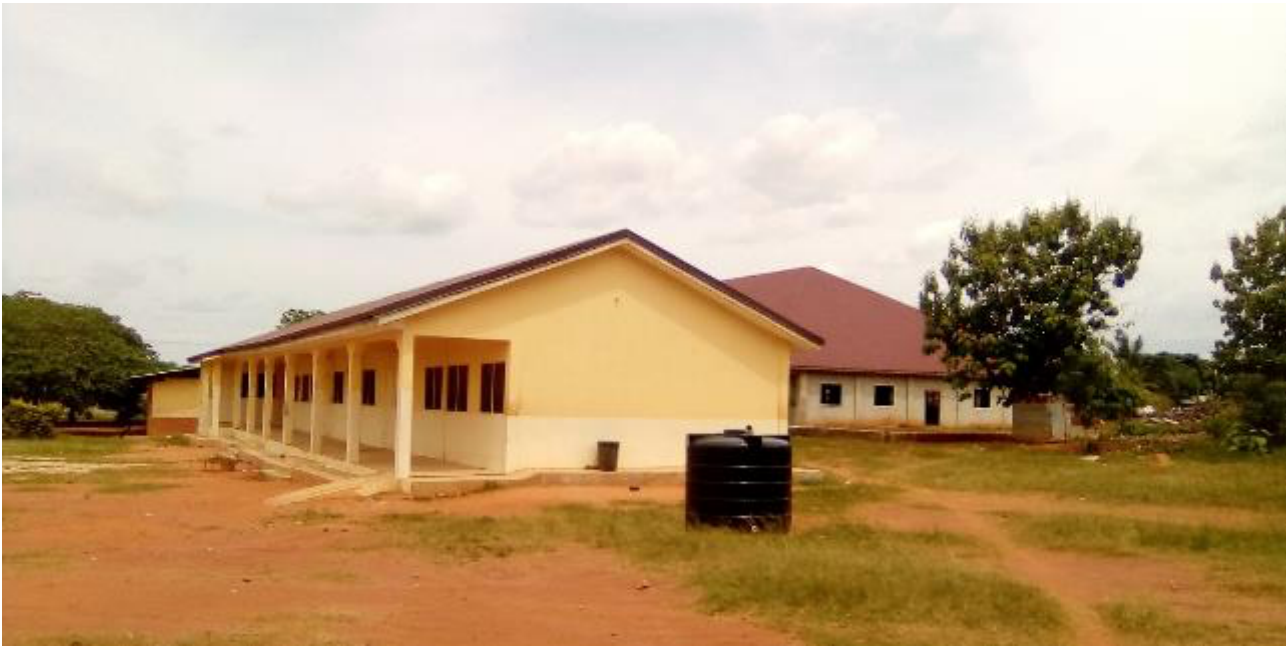
The classroom block with the tank behind it
